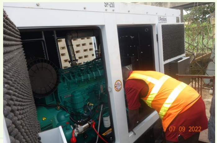
Installation of the 250KVA Perkins soundproof Generator
