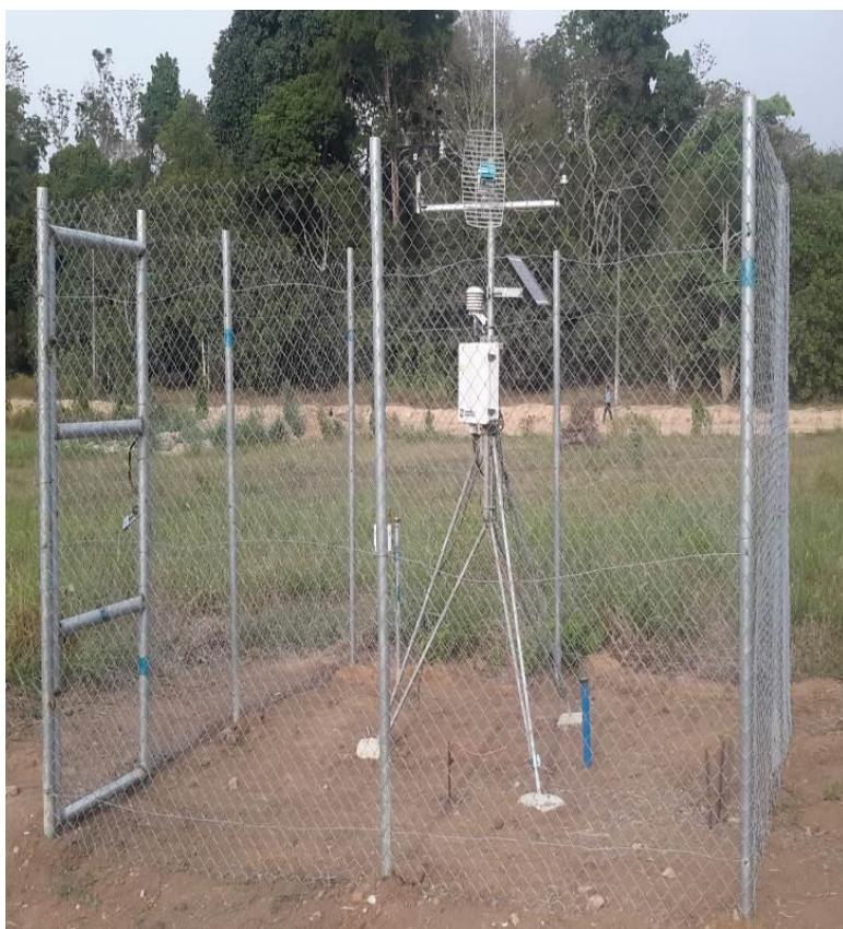
Newly Constructed Automatic Weather Station
