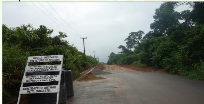
On-going road construction at the Senior Staff Quarters
