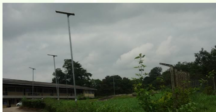
On-going solar electrification project
