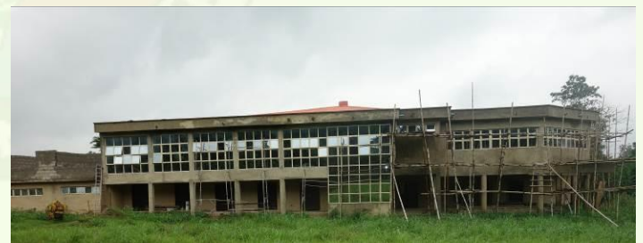
On-going 1500 capacity conference hall
