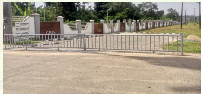
Ultramodern Perimeter Fence with Visitors' Car Park
