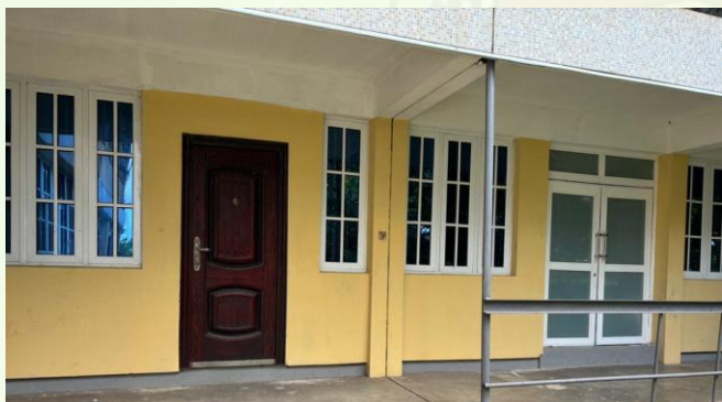
Renovated Value Addition Research Offices and Laboratory
