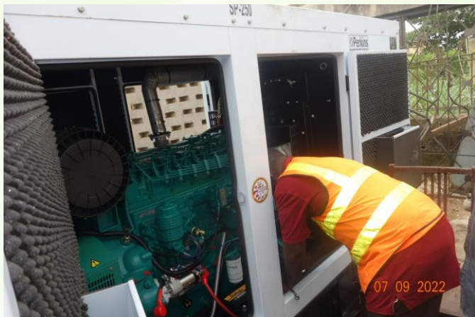
Installation of the 250KVA Perkins Soundproof Generator
