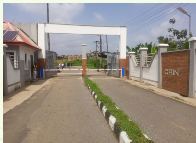
Remodelled CRIN Frontage and Gate
