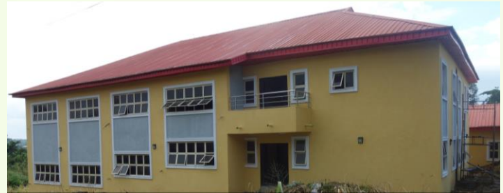
Front View of the Central Laboratory
